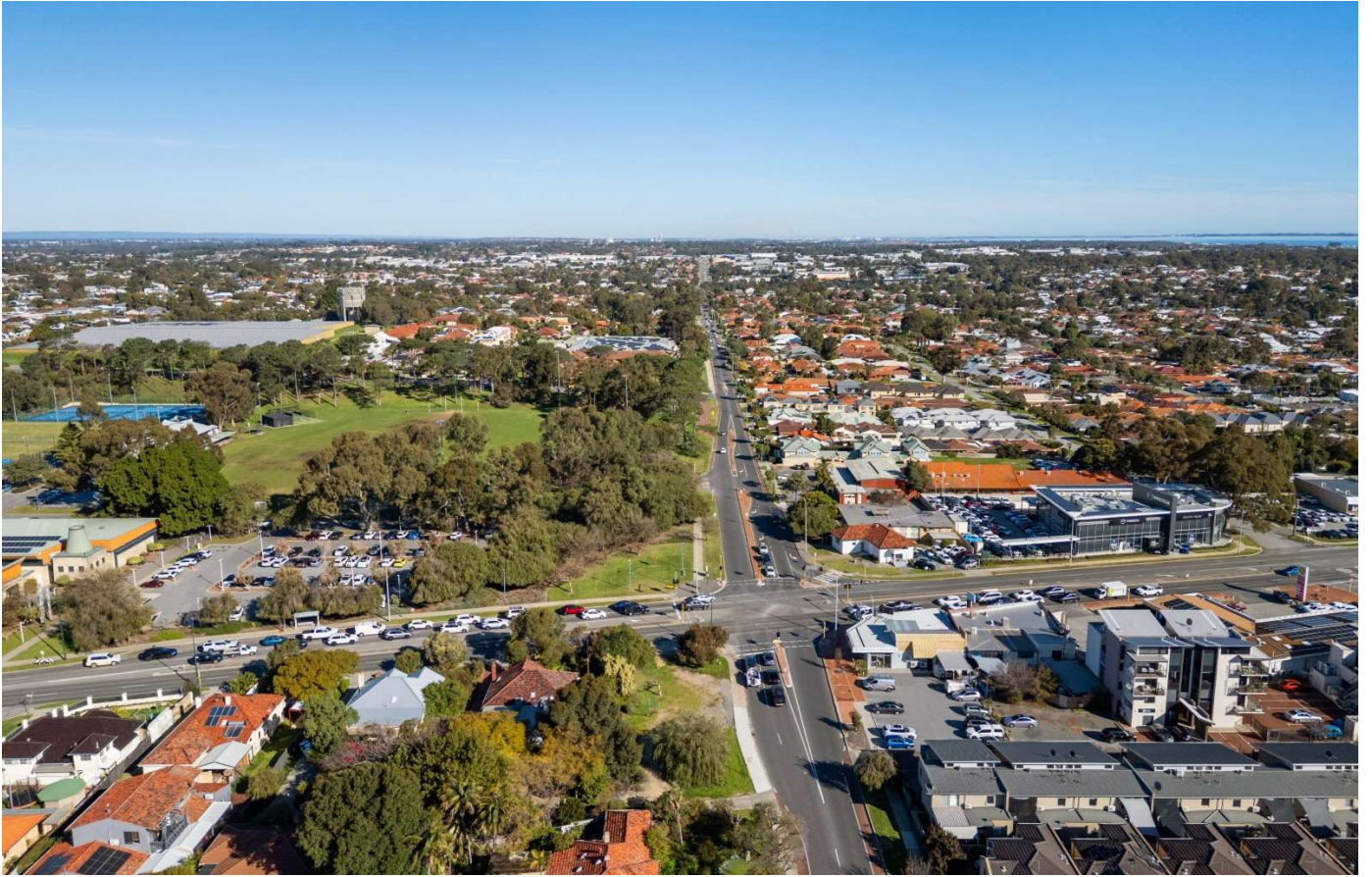
Figure 9 Photograph of broader site context facing south
