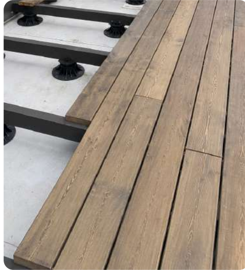
Timber Decking on Pedestals to Podium Cafe area
