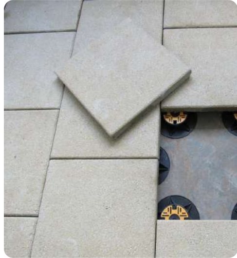
Concrete Unit Pavers on Pedestals to upper level common areas
