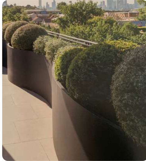
Raised Planters to Level 6 Apartment Balconies
